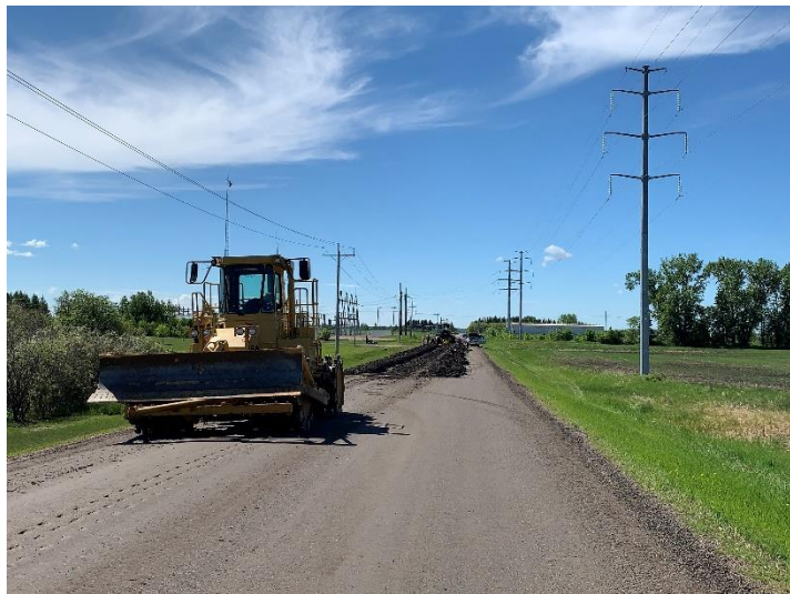
Image: Range Road 95, 2020 Construction Program
